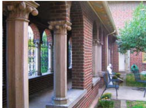
The interior courtyard of the San Damiano Friary.
